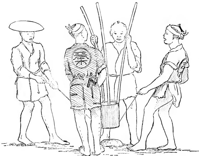
FIG. 5. — POUNDING DOWN FOUNDATION STONES.
